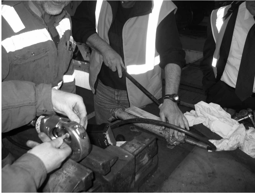
Figure 9 The hydraulic crimping tool in use at the EMU depot
