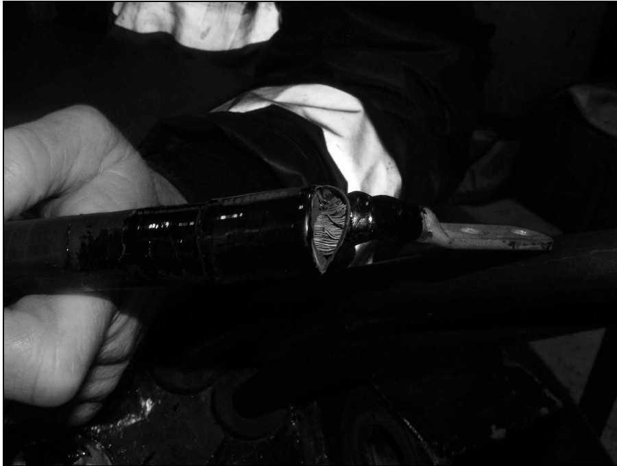
Figure 11 Recently crimped joint showing loose cable strands (Alstom Hutt)
