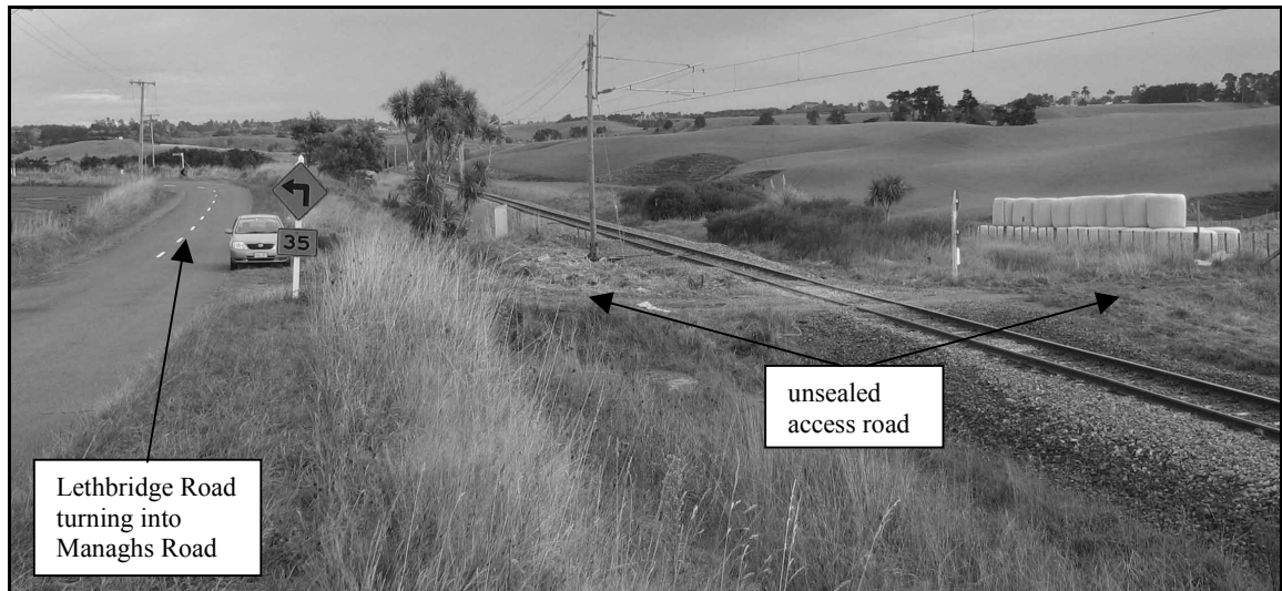
Figure 2 Overview of private level crossing and intersection with Lethbridge Road looking north
