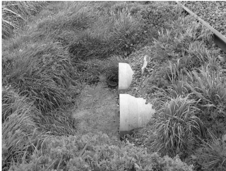
Figure 17 The replacement pipes installed at culvert 43.554
