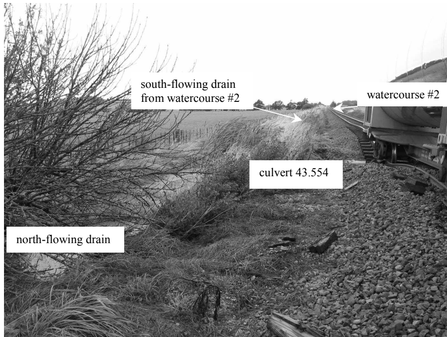
Figure 11 The drains converging at culvert 43.554
