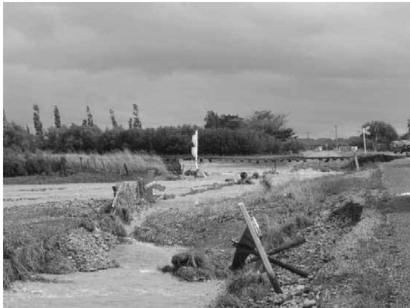
Figure 16 A section of the washed out balloon loop at Woodville
