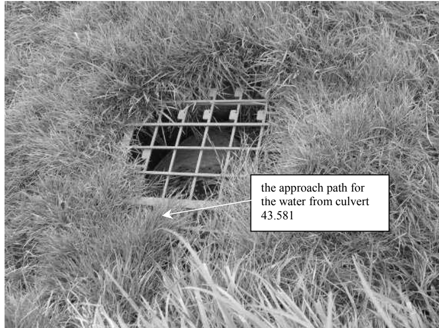
Figure 8 The sump near the exit to culvert 43.581
