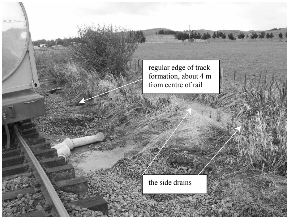
Figure 7 The edge of the track formation at culvert 43.554
