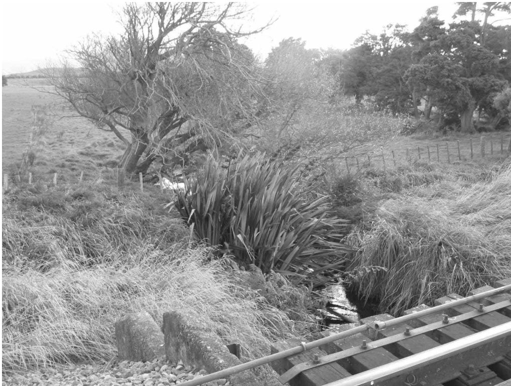
Figure 9 Watercourse #2 at Bridge 136
