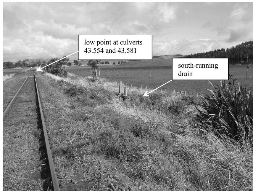
Figure 10 Looking south from Bridge 136
