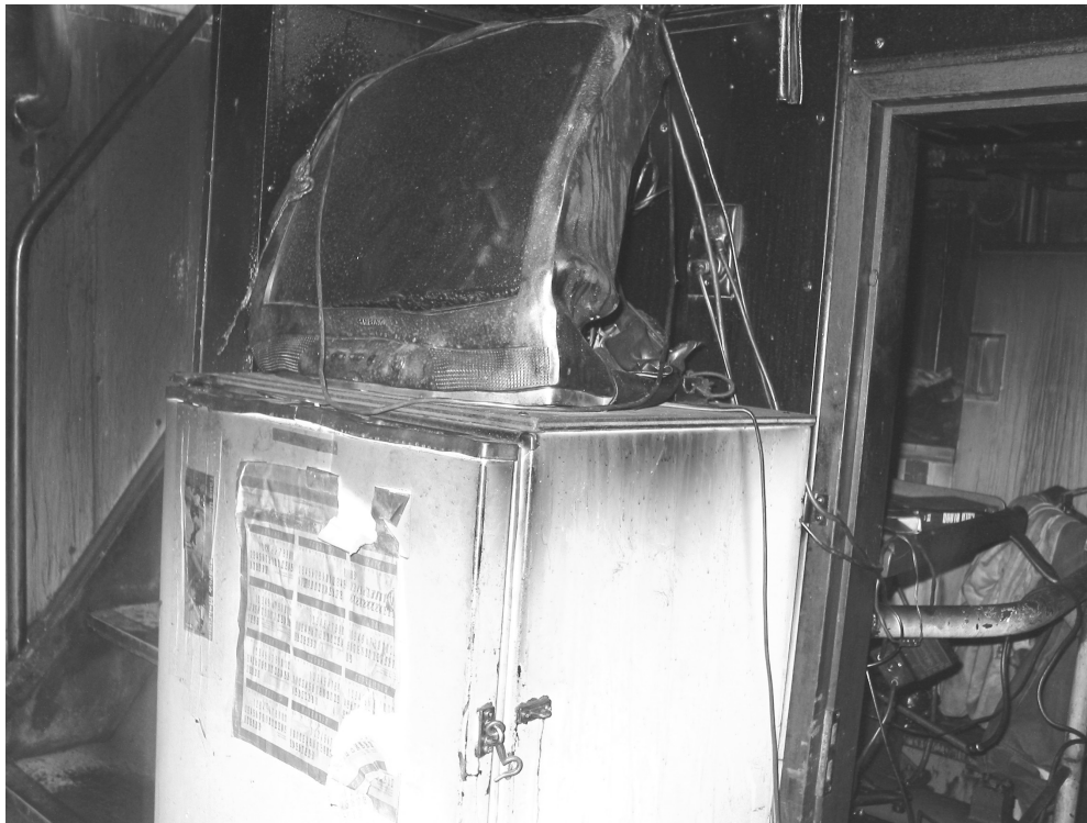
Figure 8 Refrigerator by doorway into steering gear, with melted television on top
