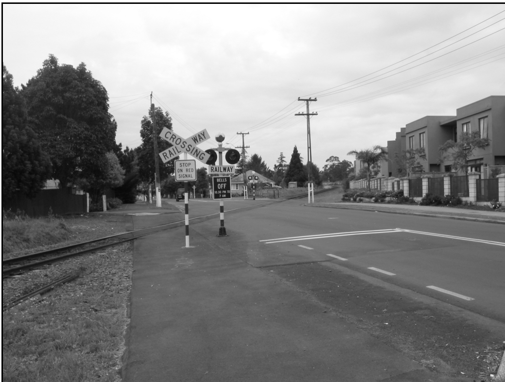
Figure 1 St Georges Road level crossing looking north
