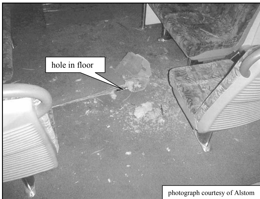
Figure 1 Damaged floor of passenger car ADL 810
