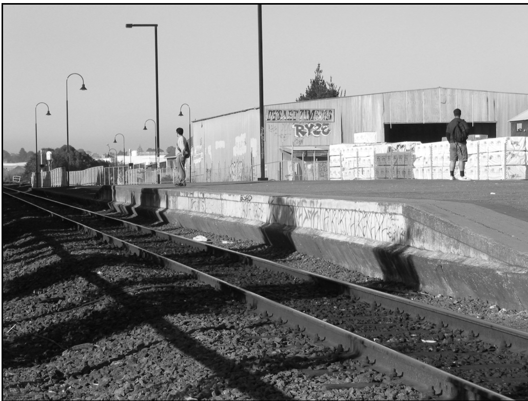
Figure 2 Down main line and platform at Glen Innes (looking south, direction of Train 3247)
