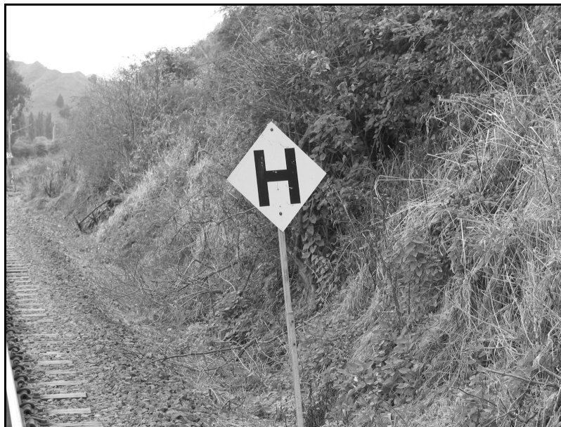
Figure 6 Temporary Heat Restriction board approaching the derailment curve
