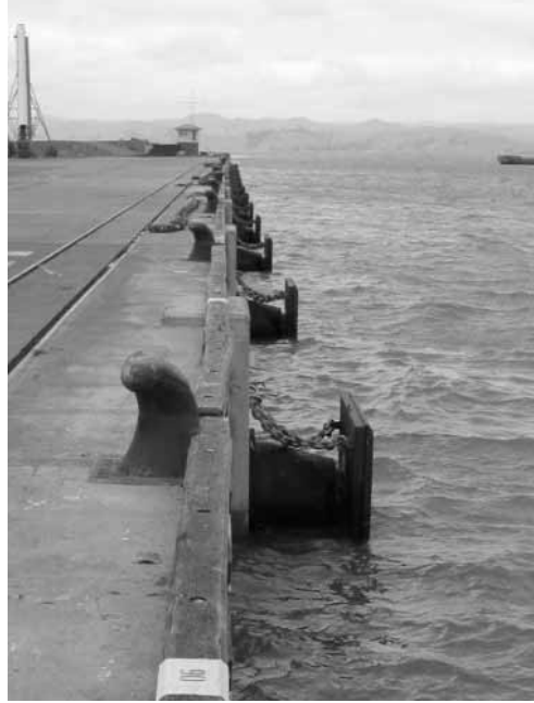
Figure 11 Fendering at number 8 wharf
