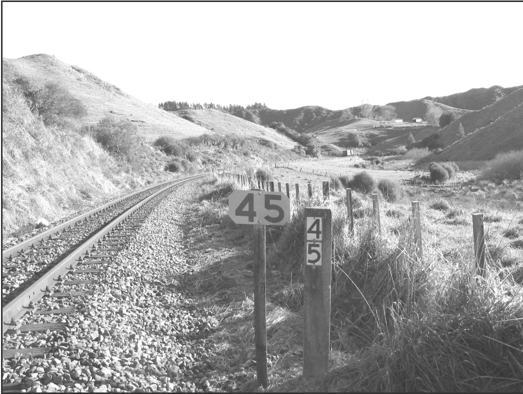
Figure 3 The 45 km/h curve warning board to the left of the 45 km metrage peg
