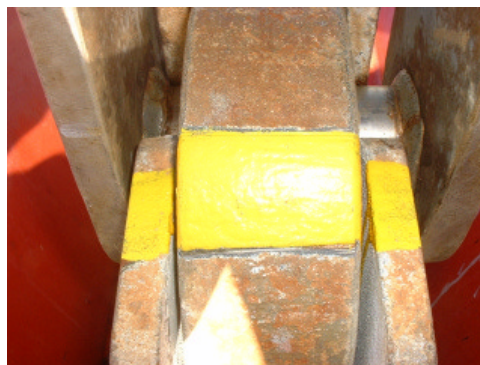
Figure 8 Markings on hook and chassis
