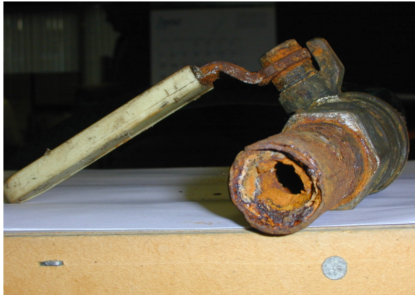
Figure 8 Internal corrosion in fractured pipe
