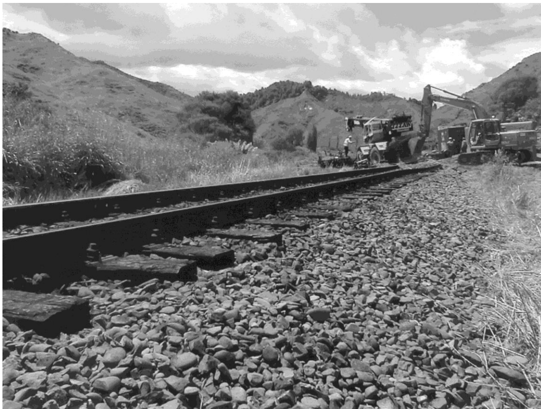
Figure 1 Typical ballast profile at 47.35 km SOL
