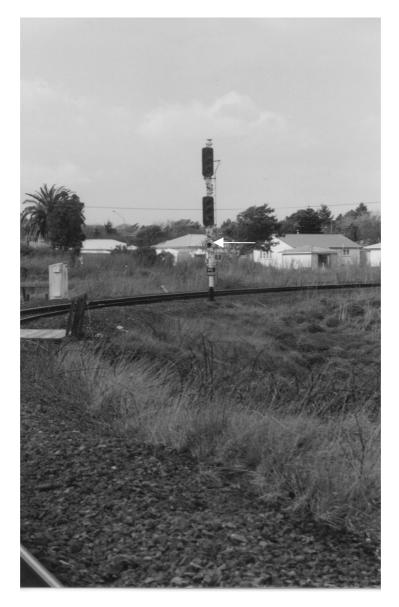
Figure 2 Signal 4R from about 200 m away. The low speed light unit is arrowed.
