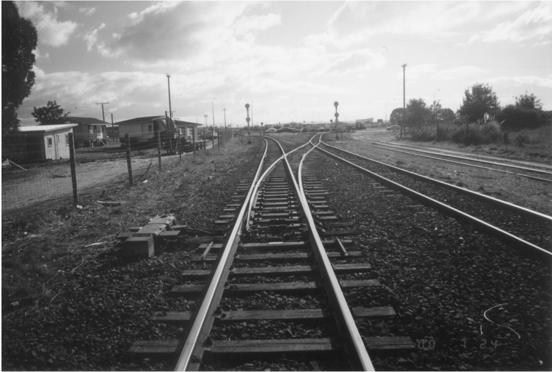
Figure 2 View looking north showing the intended route of Train 378 (to the left) and the actual route taken to the right, with SH 2 level crossing in the background
